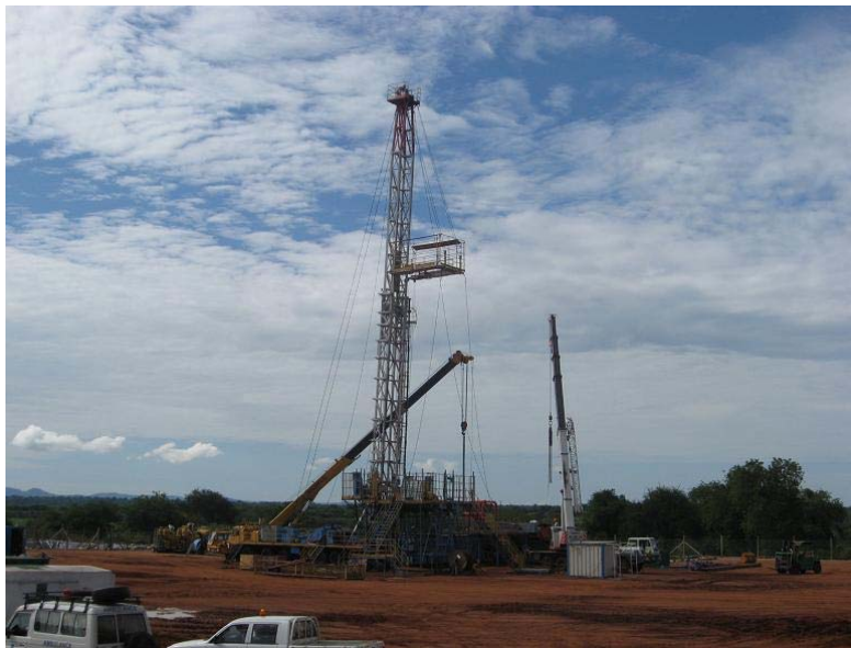
Figure 1- Arrival of MBU-125 land rig onsite.
